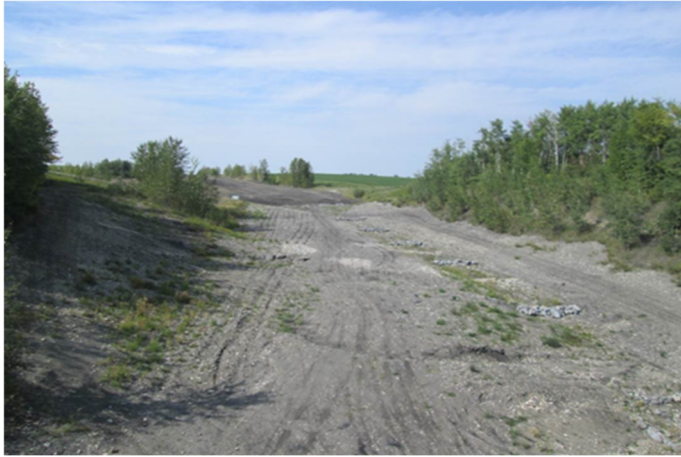
Figure 2: Looking north, drainage ditch check dams
