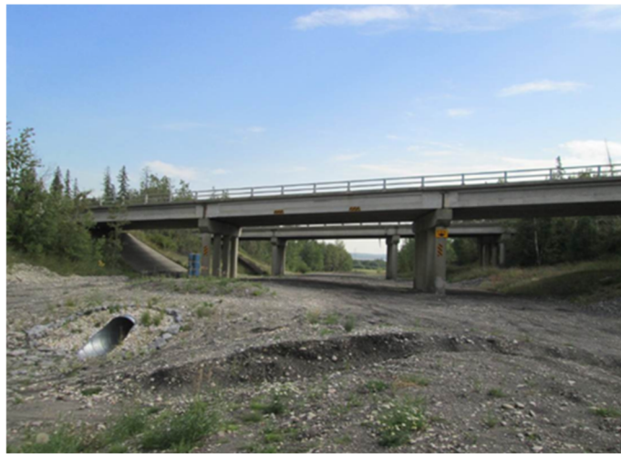
Figure 4: Looking south, drainage culvert inlet
