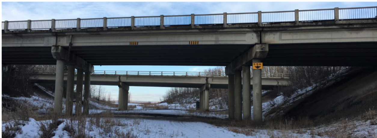
Figure 7: Looking north, vertical clearance beneath the existing bridges posted at 6.9 m
