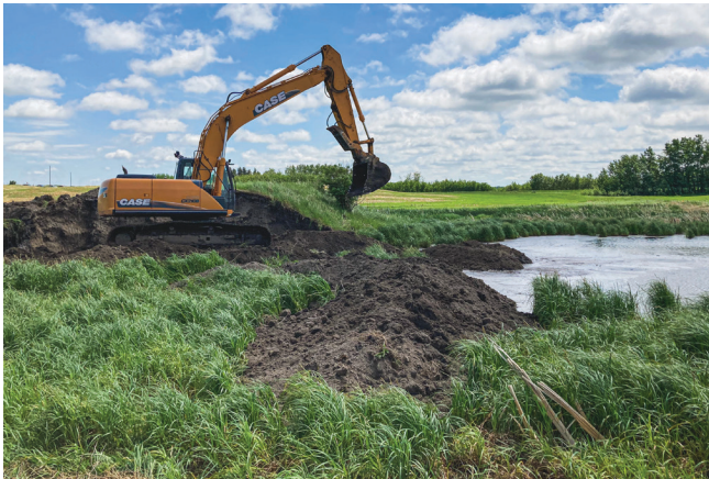
Recontouring a historical dugout to restoring a natural wetland.
