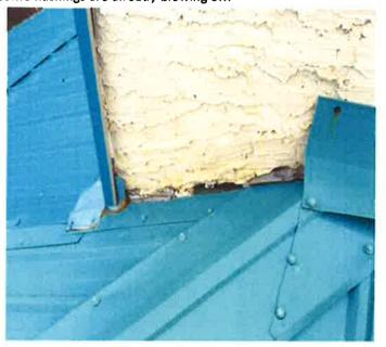
Here are some example of recent projects of mine with similar details using the proposed new system. They were designed to last 50+ years. No exposed fasteners, 24" lapped panels and thermal expansion high wind clip system with custom flashings. A system that does not rely on sealant and is fabricated onsite with the correct tools. It is a structural system and by all accounts the best option for your re roof.
