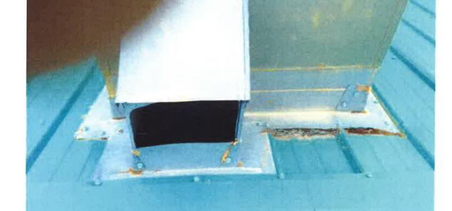
All of the roof penetrations are installed incorrectly. Water is forced directly into the lower side of the improperly lapped panels. They rely on caulking to create a water tight seal and can never be repaired. Caulking as a sealant has a maximum life expectancy of 1 year for this application before it starts to fail. These have been temporarily repaired several times already.
