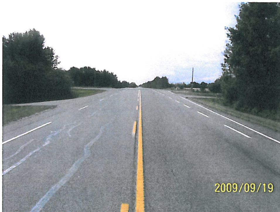
PHOTO # 2 – Viewing South from north of the intersection of Hwy. 770 and Parkland Drive. A Type II intersection treatment exists, with the tapers slightly longer on the east side .
