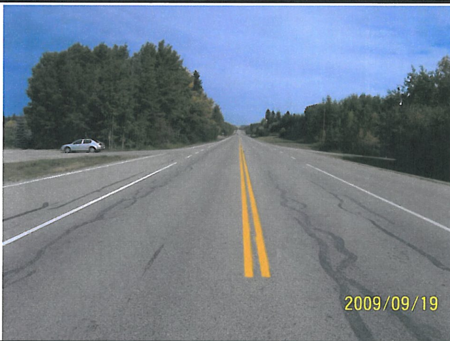
PHOTO # 4 – Viewing North from the Hwy. 770 & Parkland Drive intersection. There is more than 600m of sight distance available. A road/approach exists on the left.
