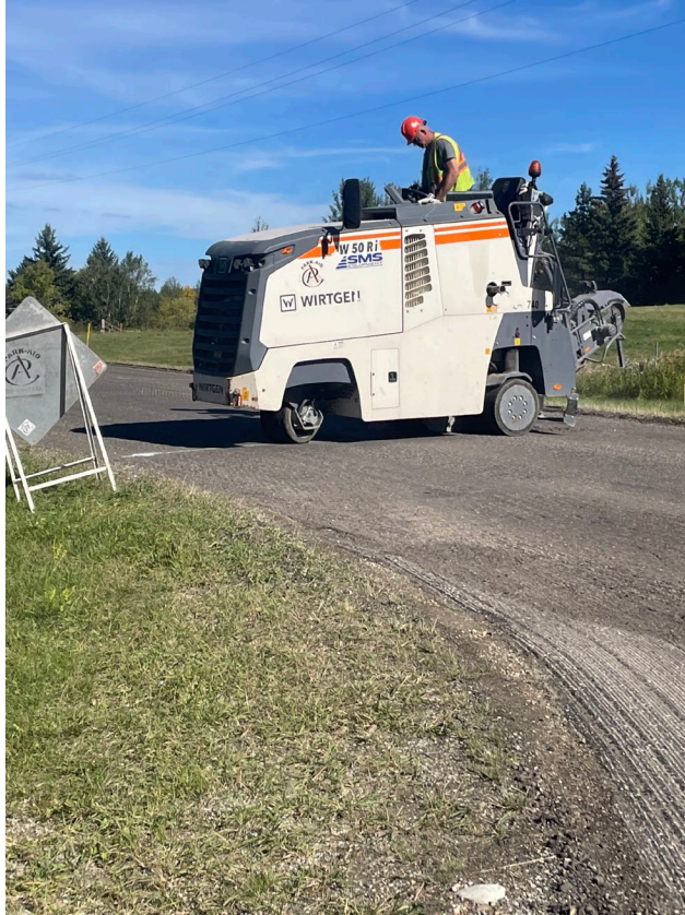
Grading deeper depth in areas where we have transverse cracking on the roadway
