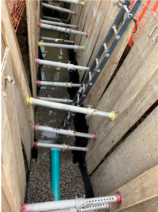
View of the bottom of a trench within Osprey Subdivision. New Sanitary pipe on sand/aggregate bedding
