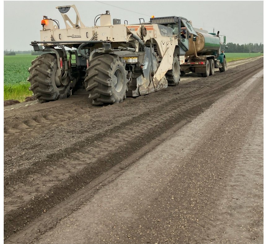
Water Truck and Roadway Reclaimer pulverizing the existing road surface.
