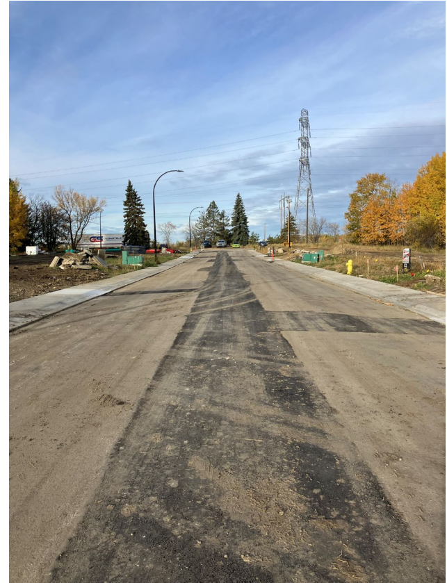
Osprey post sanitary line repairs
