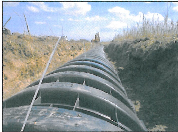
Figure 4-5 Installation of Chambered Infiltration Trench
